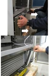
Remove the electrical panel locking screw.
