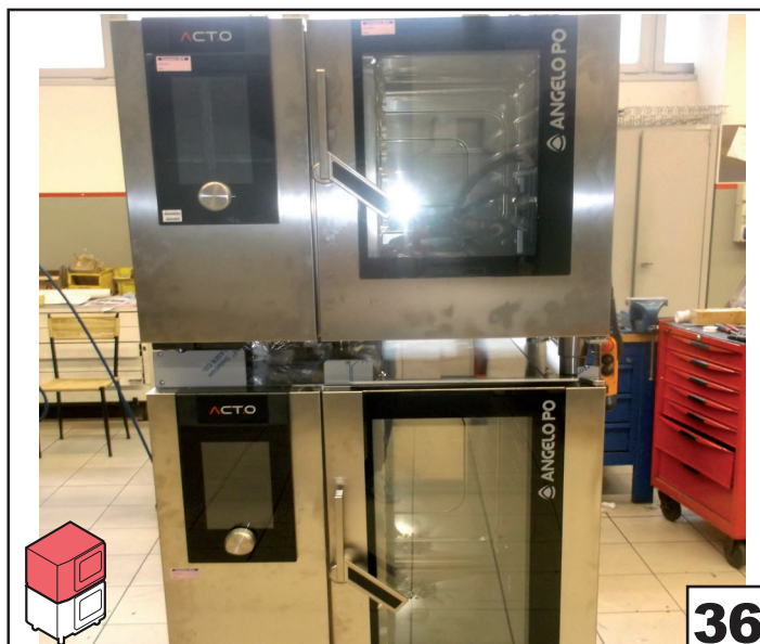
36 Place the top oven using the feet references on the base supports
